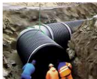
Welded joint
